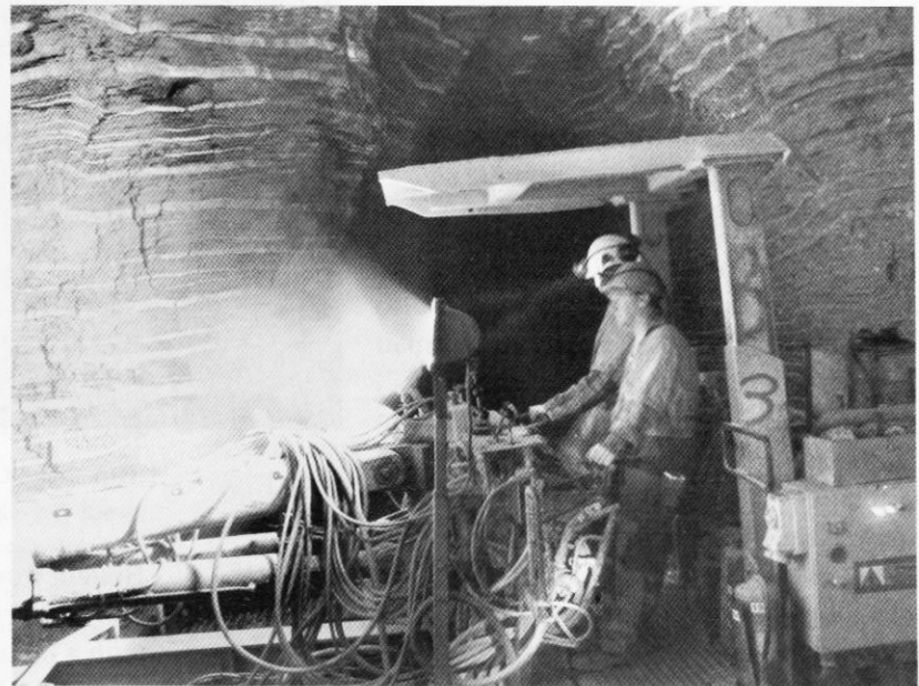
Birkshead Gypsum Mine - boring rig - picture Joep Orbons
